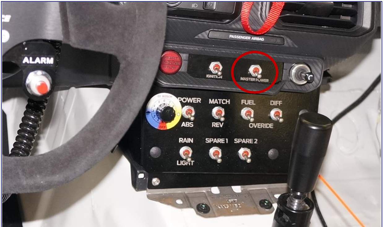
Interior Master Power Electrical Switch
