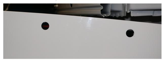
Open the 1/8" pilot holes in the bracket to  $1\ 1/8"$
