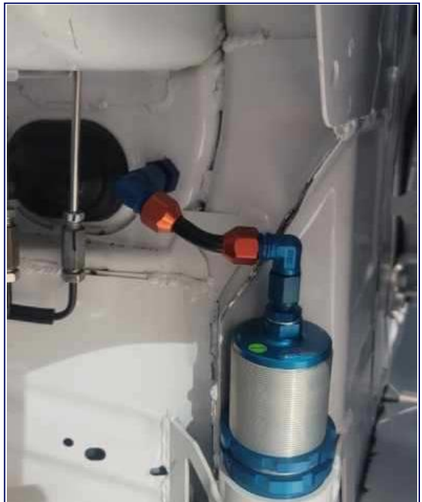
Front Air Jack / Bulkhead Connection Driver Side
